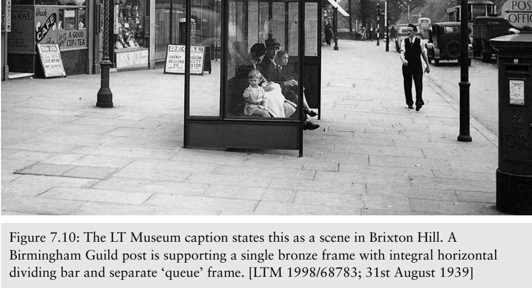
Figure 7.10: The LT Museum caption states this as a scene in Brixton Hill. A Birmingham Guild post is supporting a single bronze frame with integral horizontal dividing bar and separate 'queue' frame. [LTM 1998/68783; 31st August 1939]
