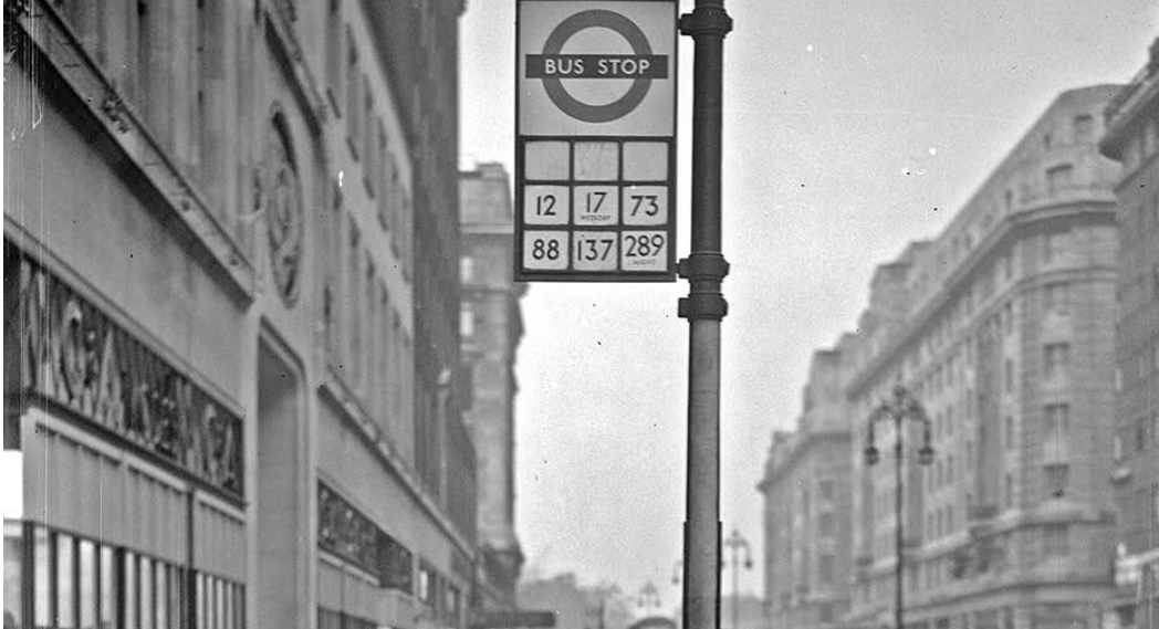
Figure 7.11: This post at Marble Arch has three fixing points though the spacing of them has the lower two close together. Evidence of wartime blackout painting can be seen on the post. [LTM 2009/12455; December 1940]
